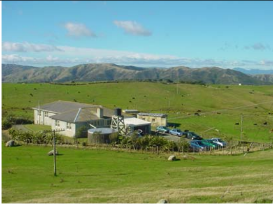
Quartz Hill buildings, looking towards Mt. Kaukau
