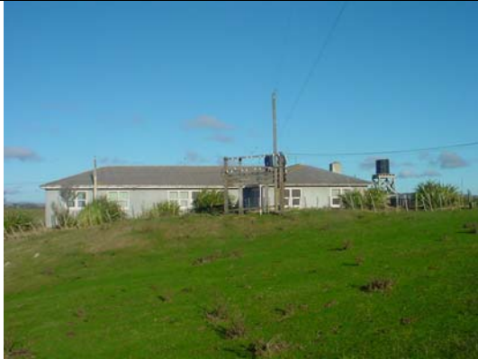
Western side of Quartz Hill building
