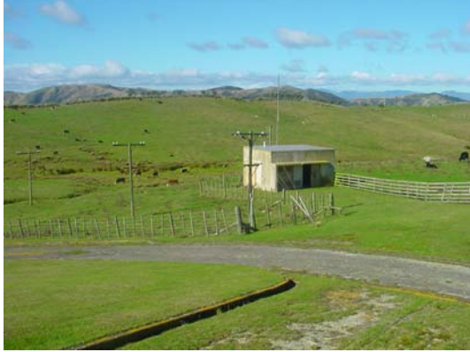
Old diesel hut in foreground, looking northeast
