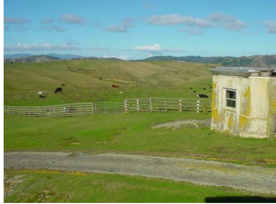
The old original station building; now derelict
